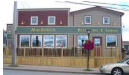
Newly Renovated Business Storefront
